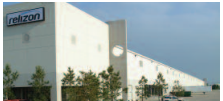
This attractive 250,000 sq.ft. distribution center was completed in only 94 days!
