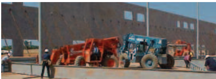
Modular sections are assembled quickly and safely on the ground.
