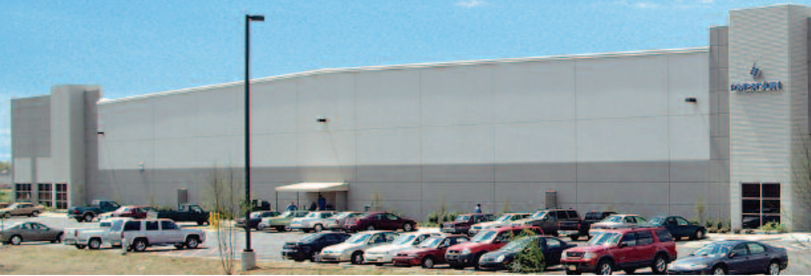
This spacious one million square foot warehouse was enclosed in just 34 days.
