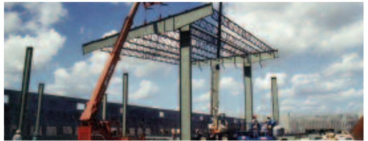
Entire bay assembly can be lifted in one piece.
