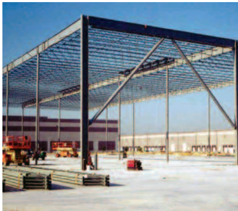
The Long Bay System provides bay spacing up to 65 feet; the largest column-free spaces in the industry.
