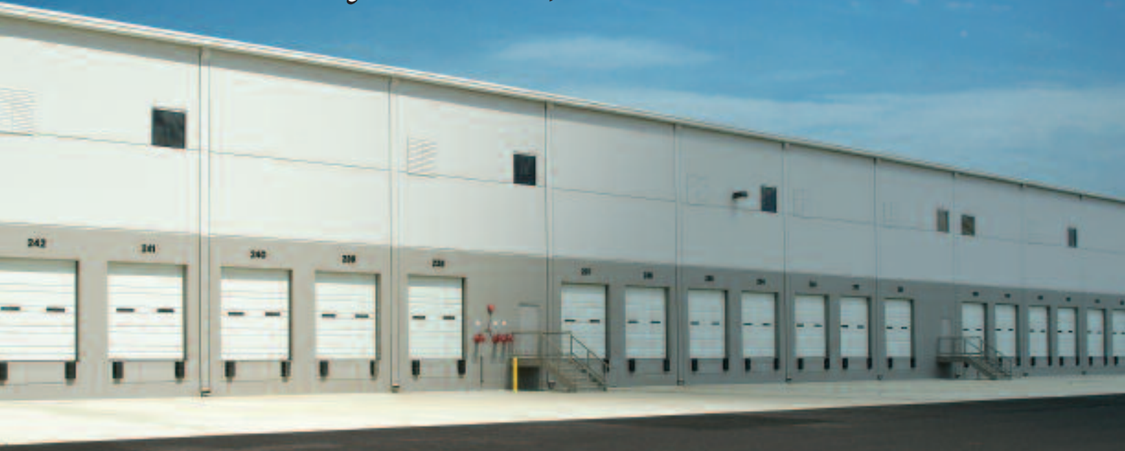
The Long Bay System was used in the construction of this spacious, one million-sq.ft. warehouse.
