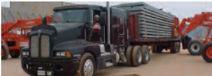
Complete load of frames is unloaded using 4-point pickup method.
