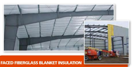
Laminated fiberglass insulation is a widely used form of insulation. This type of insulation blanket is used in a variety of installation methods; however, it is typically installed between the structural steel or wood and the roof or wall material.
