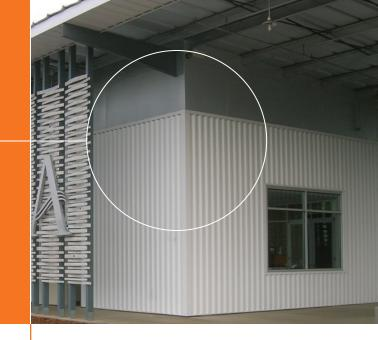
The **7.2 Insul-Rib**<sup>TM</sup> insulated metal wall panel combines a traditional 7.2 rib panel design with a polyurethane foam core. This widely used profile is available as an insulated panel in various thicknesses.
