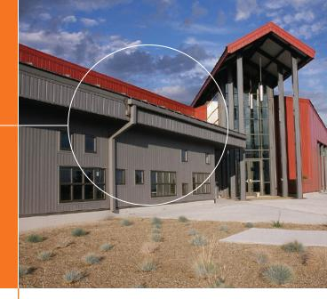
The ribbed profile of the **Fluted** insulated metal wall panel provides bold vertical lines complementary to almost any commercial or industrial building. Inverted ribs in the profile enhance the high-tech industrial look.
