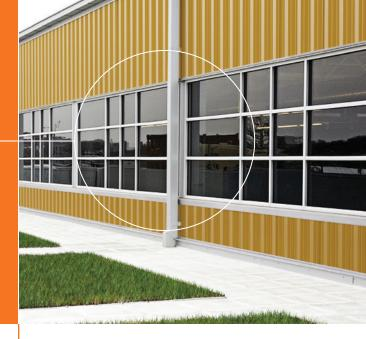
The versatility of the LS-36™ insulated metal roof and wall panel offers a multitude of design options. The deep ribs create an even-shadowed appearance and the overlapping, through-fastened joint allows for quick installation.
