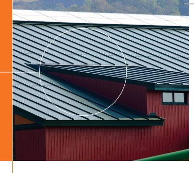
The **CFR** panel is an insulated metal standing seam roof panel, combining durable interior and exterior faces with a polyurethane foam core.
